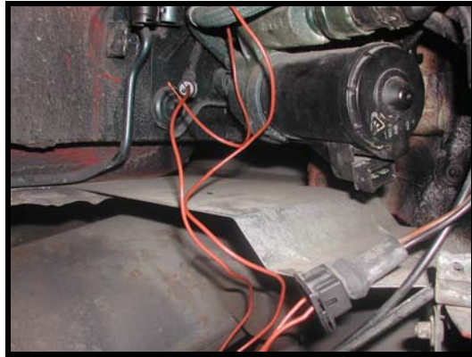
Picture of Jumper Leads connecting the High Pressure Pump power supply to the Magnetic Lock Valve female power connector
