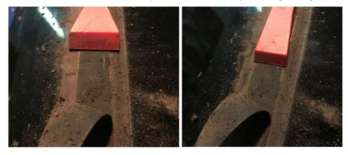
To remove the glue residue I used cloths, acetone and a lot of elbow grease.....
